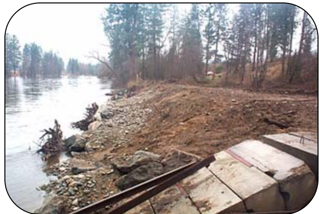
Streambank Stabilization on Kettle River
